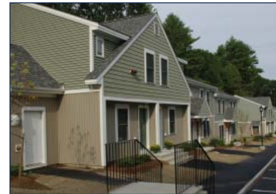
Parmenter Place: Concord, NH Sponsor: Concord Housing & Redevelopment Authority Units: 25 family Architect: Steve Burnell Permanent lender: Merrimack County Savings Bank Construction lender: New Hampshire Housing General contractor: North Branch Construction Construction jobs saved or created: 33
