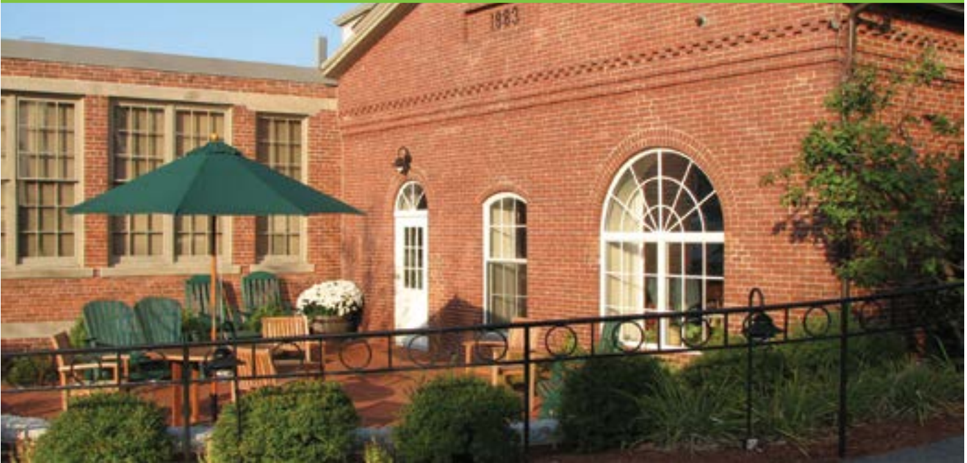
Milford Mill, Milford
